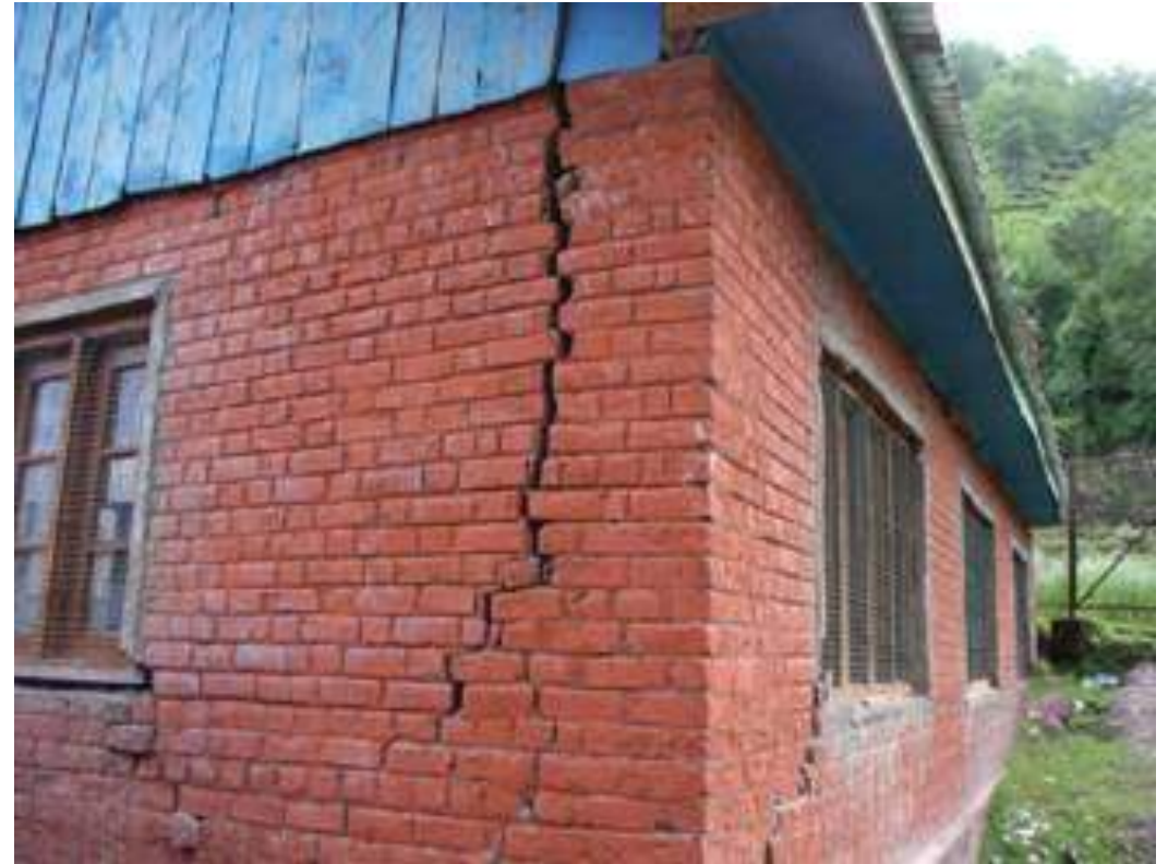
Damage due to poor wall to wall bonding
