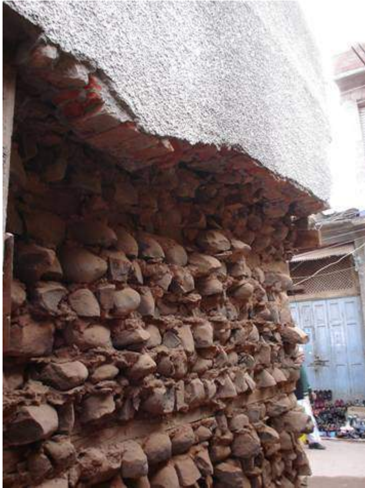
Need for Installing Bond Element
