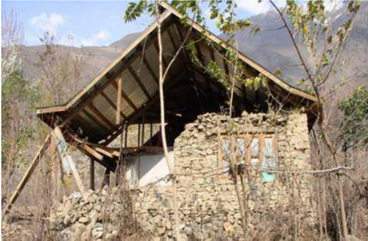
Roof damaged due to inadequate tying.
